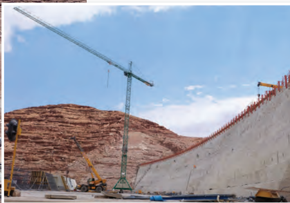
Salini Impregilo will use more than 1 million m 3 of concrete will be used in the construction of the Neckartal dam
